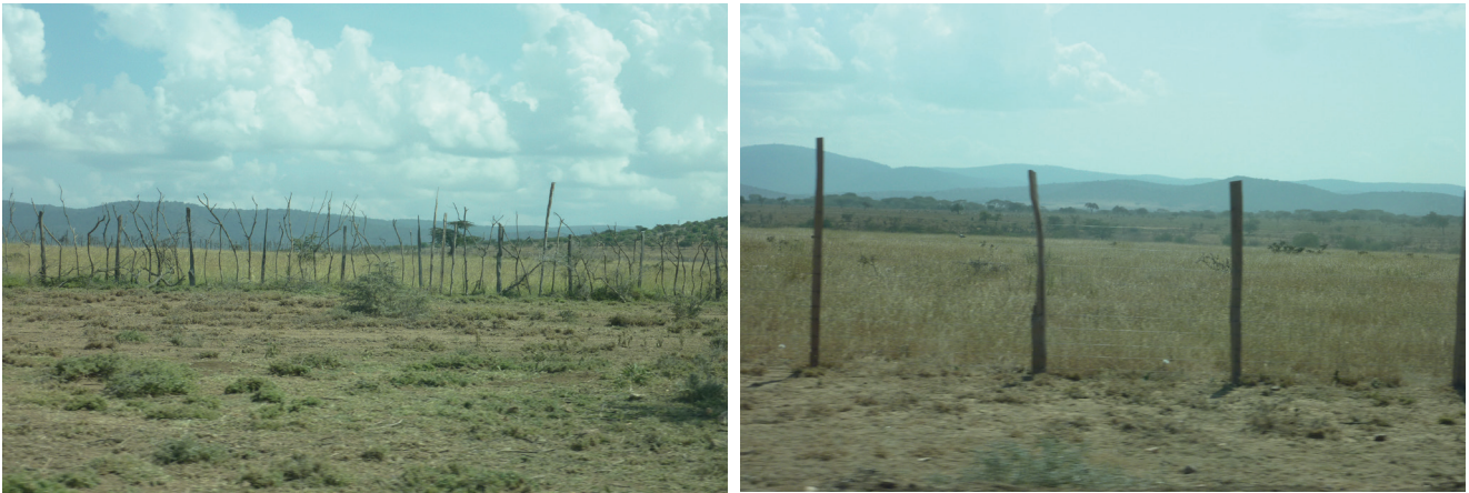
Figure 7. Fencing of Land by Individuals in Naroosura Group Ranch Restricting Collective Access
